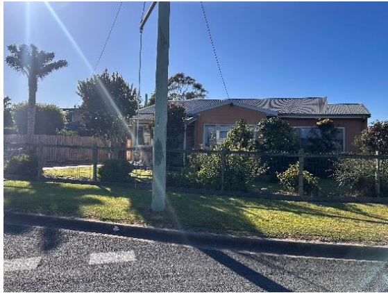
Photograph 2 – Subject site at 31 Ferndale Parade, Lakes Entrance.
