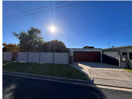
Photograph 22 – Neighbouring property adjoining the western boundary at 33 Ferndale Parade, Lakes Entrance.
