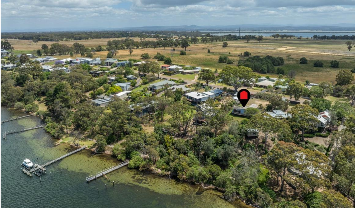
Subject land looking north (Source: King & Heath)
