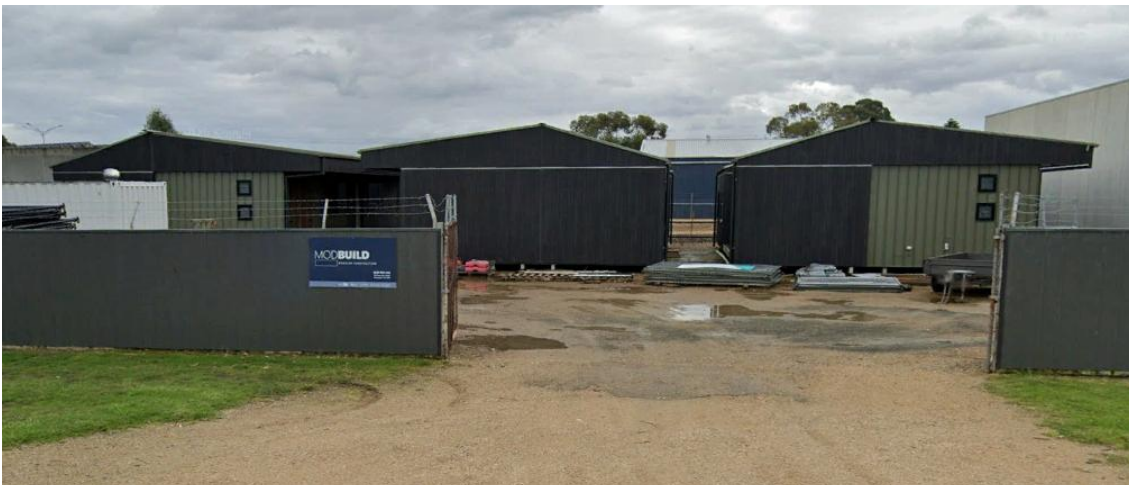
Construction Company (90 Dalmahoy Street) looking north from Dalmahoy Street
