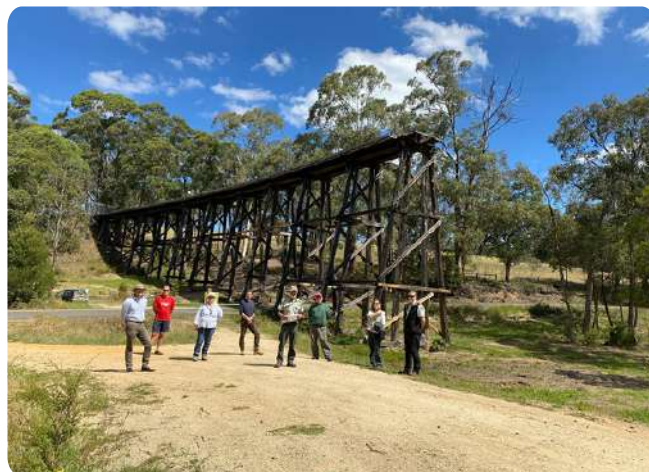
Wairewa Road Railway Bridge, Wairewa
