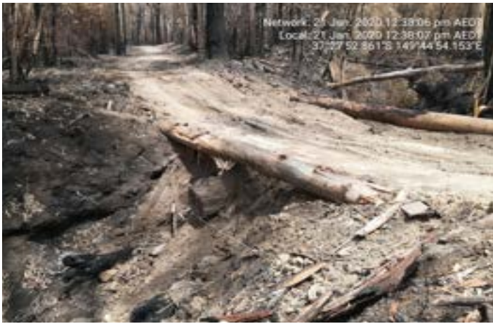
Fairhaven Road Little River Tributary Bridge: before.
