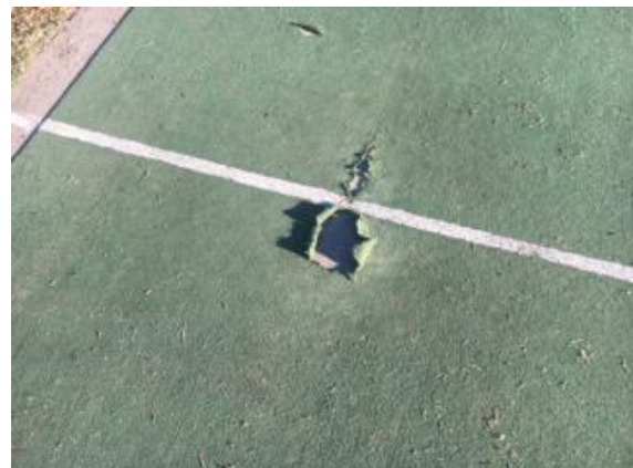
Picture 6 Damage to pitch surface
