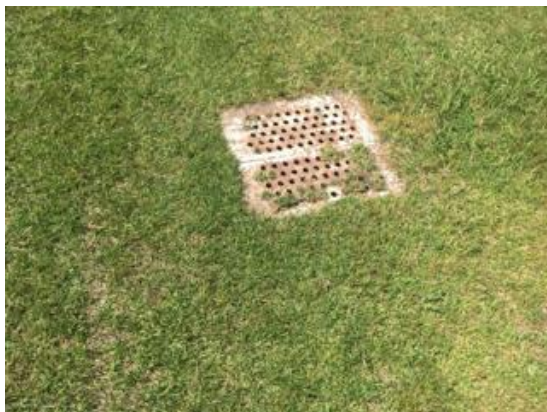
Picture 5 Drainage pit
