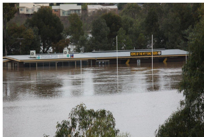
Figure 4: Wy Yung Recreation Reserve Sports Pavilion (June 2012)
