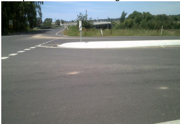
Completed Wuk Wuk bridge
