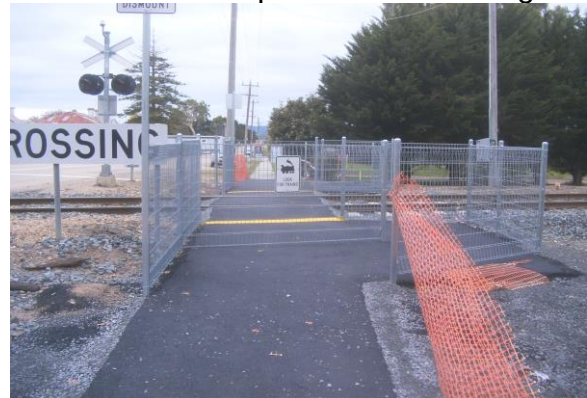
Lindenow South pedestrian crossing
