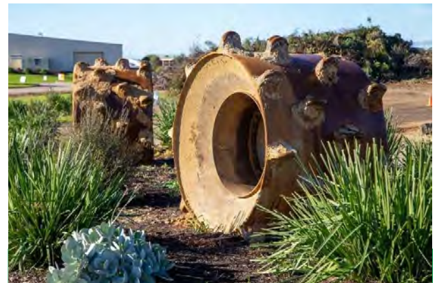
Progress continues for the Organic Waste Processing facility development at the Bairnsdale Landfill.
