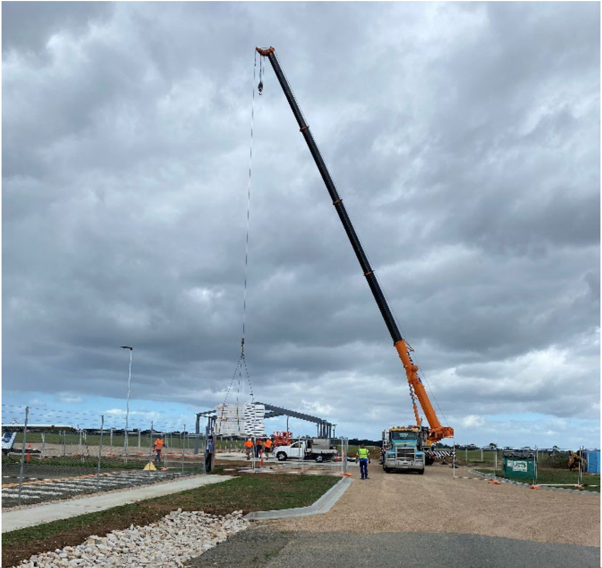
Progress at the Air Ambulance Transfer Facility at Bairnsdale Airport - January 2025.
