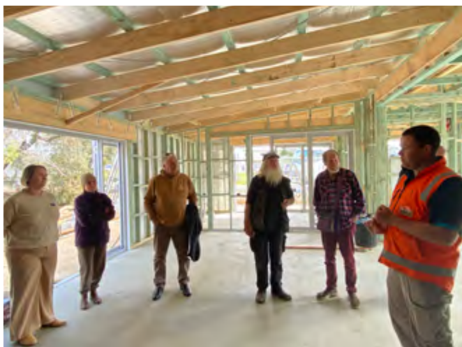
Project Supervisor, Dale Stephenson, discussing the upgrades to the Mallacoota Hall during a Councillor visit.
