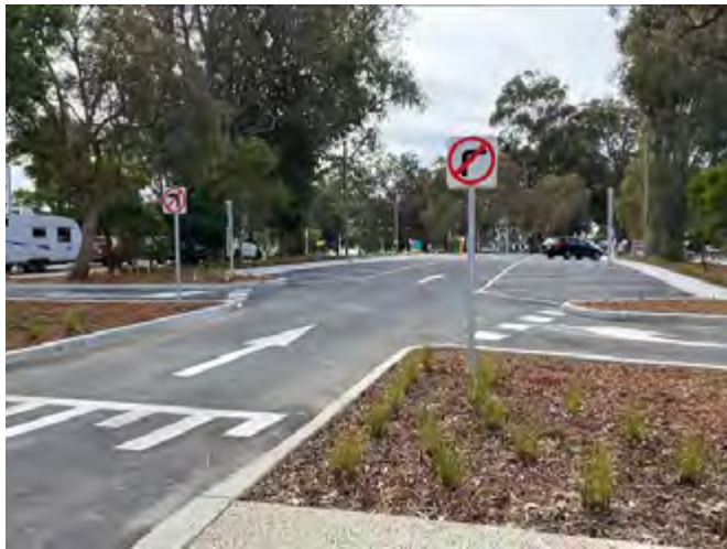
The Maccacoota Streetscape upgrade has made the town centre safer and easier to move through.
