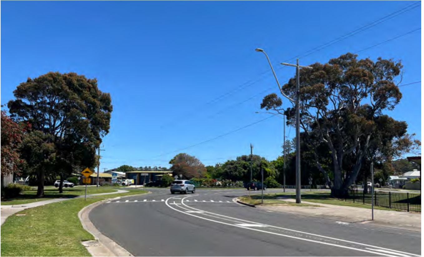
Road safety works in Church Street, Lakes Entrance.
