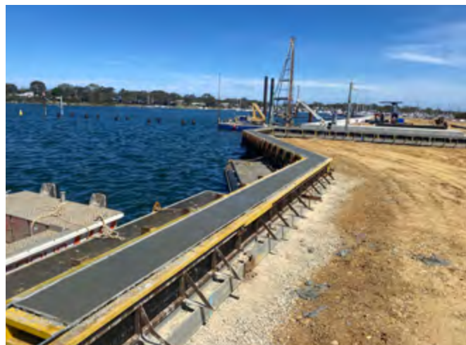
New seawalls, jetty berths, a service jetty, commercial boat ramp, drainage infrastructure and improved public access areas under construction at the Slip Road Maritime Precinct in Paynesville.
