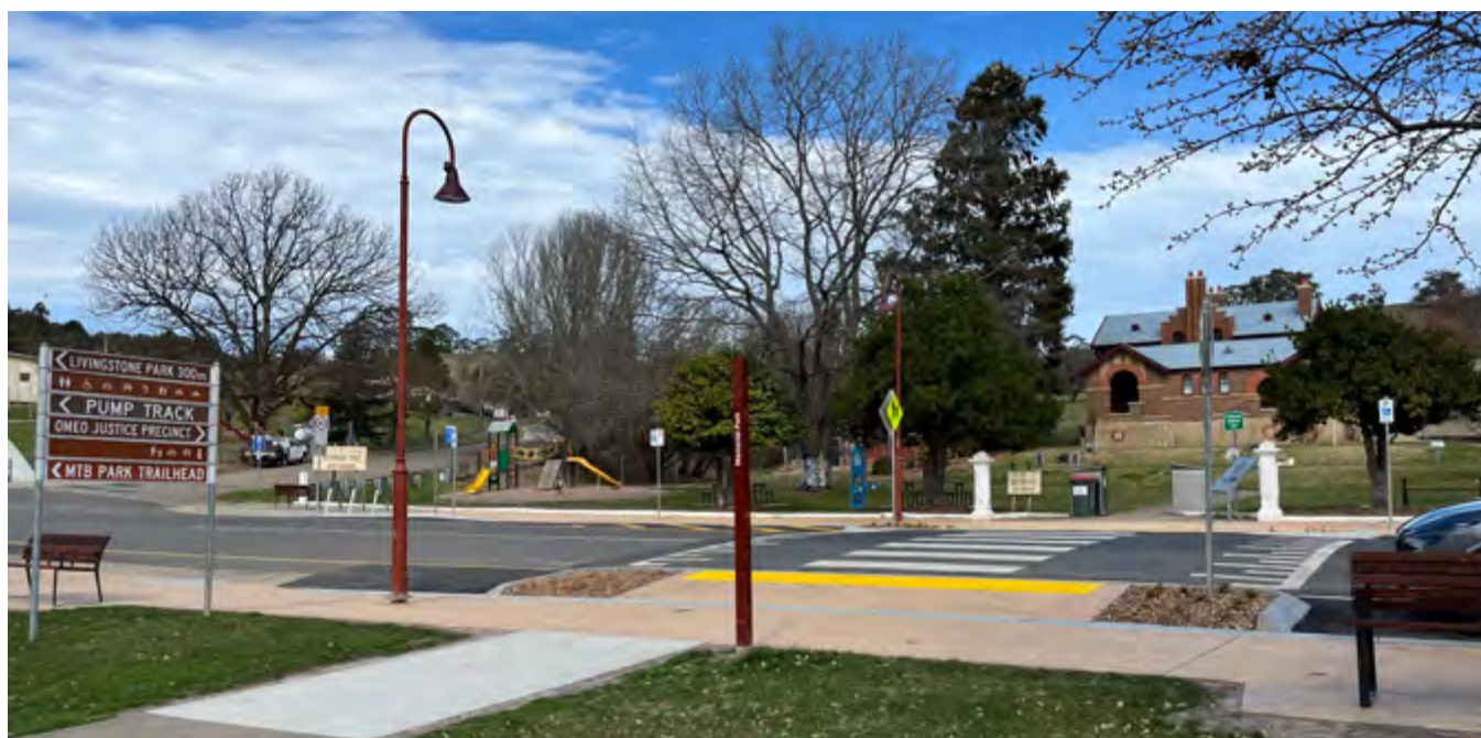
Omeo streetscape revitalisation works were completed in July.
