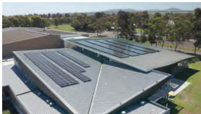
Stage one of the Bairnsdale Aquatic and Recreation Centre roof renewal was completed.
