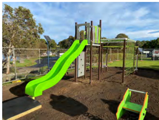
A new playground installation at Harry Clues Reserve in Johnsonville.
