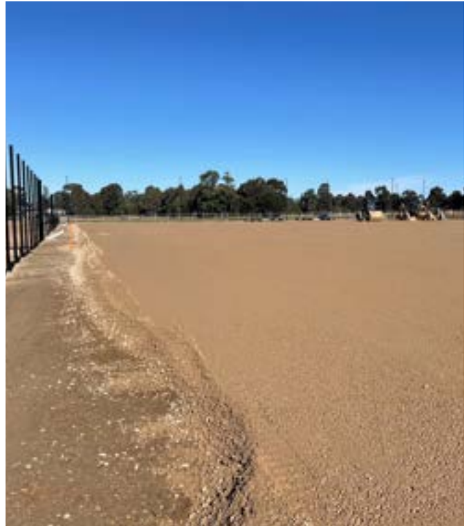
Foundations for the hockey pitches at the WORLD Sporting Precinct.
