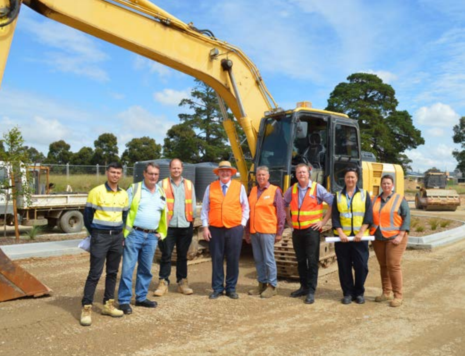
Minister for Local Government, the Hon Shaun Leane joined Mayor Cr Mark Reeves, Deputy Mayor Cr Arthur Allen, CEO Anthony Basford and our project officers and contractors for a tour of the works underway at the WORLD Sporting Precinct Redevelopment in Bairnsdale.
