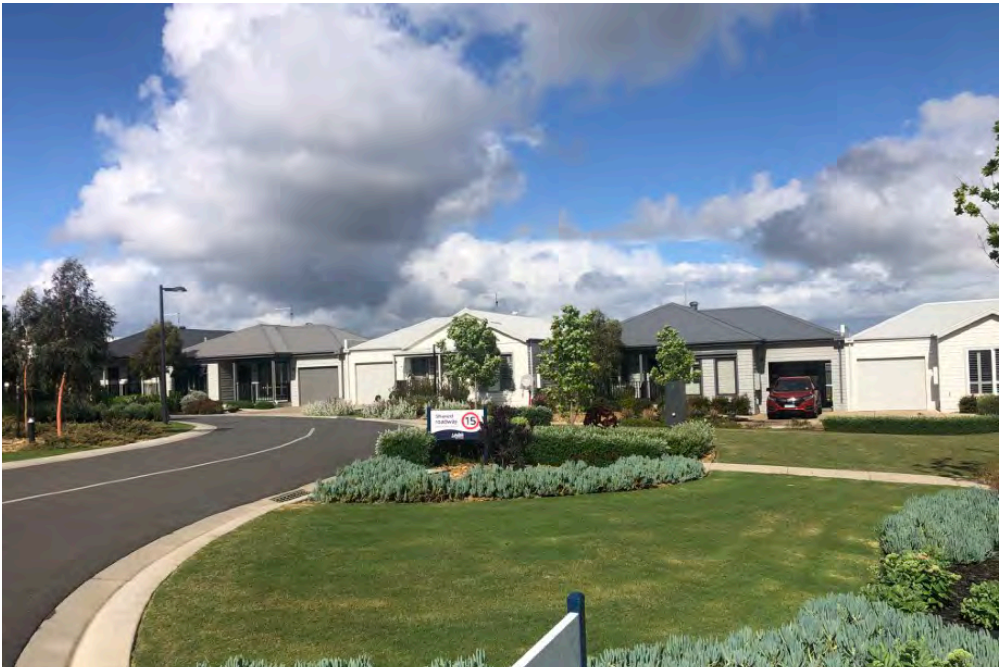
Figure 5. Typical Residential Village streetscape
