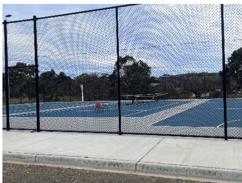
Figure 49: Omeo Netball and Tennis Courts
