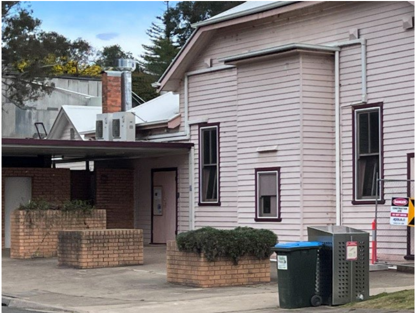
Figure 44: Swifts Creek Hall Public Toilets
