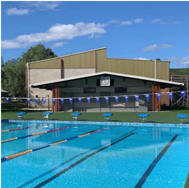
Figure 51: Swifts Creek Memorial Pool
