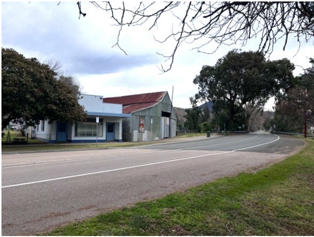
Figure 38: Great Alpine Road looking north to the Swifts Creek Bridge
