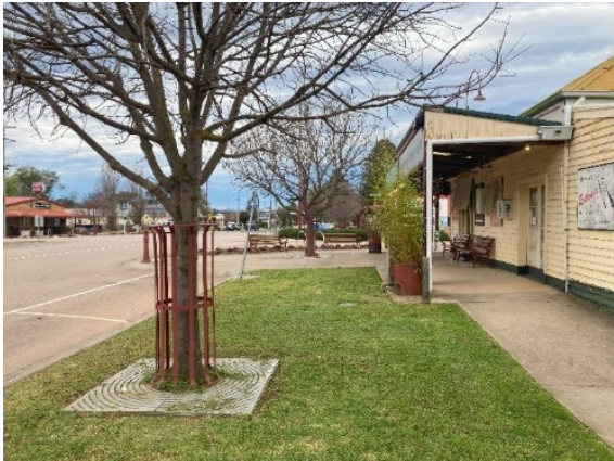
Figure 33: Redundant tree protection
