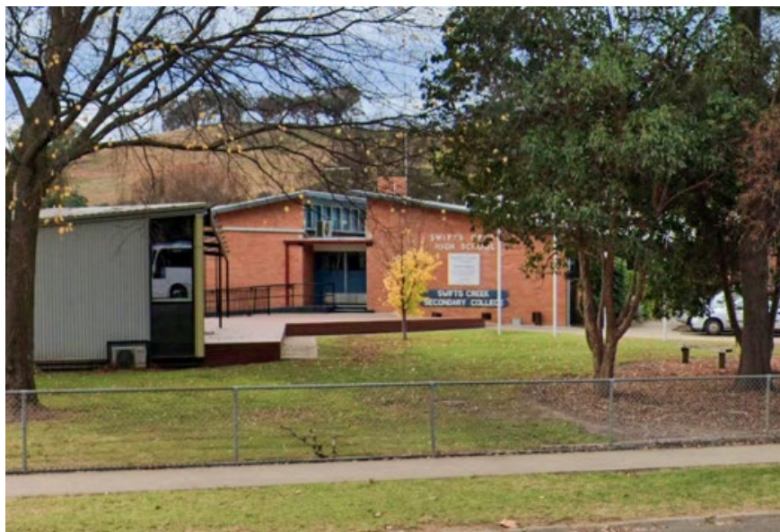
Figure 42: Swifts Creek P-12 School Tambo Campus
