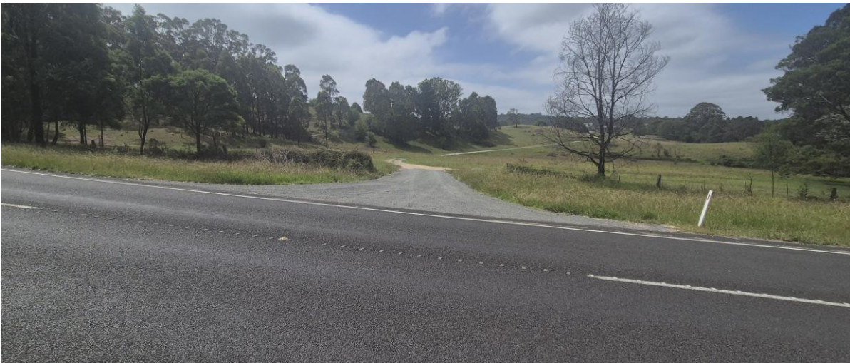
View towards subject land and existing access from Metung Road
