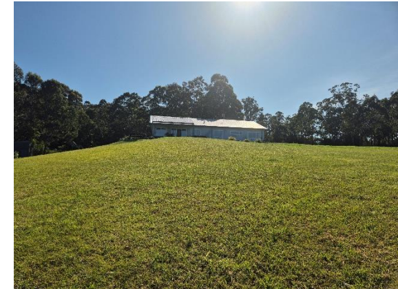
Photograph 6 – Proposed Lot 1 facing east.
