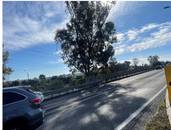
Photograph 15 – Main Street facing east – Mitchell River Bridge.
