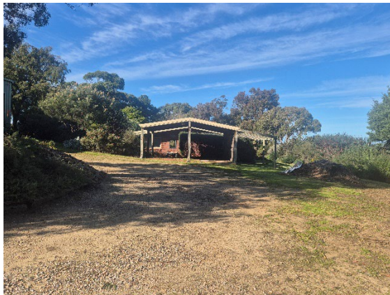
Photograph 3 – Existing dwelling on proposed Lot 1, facing south.
