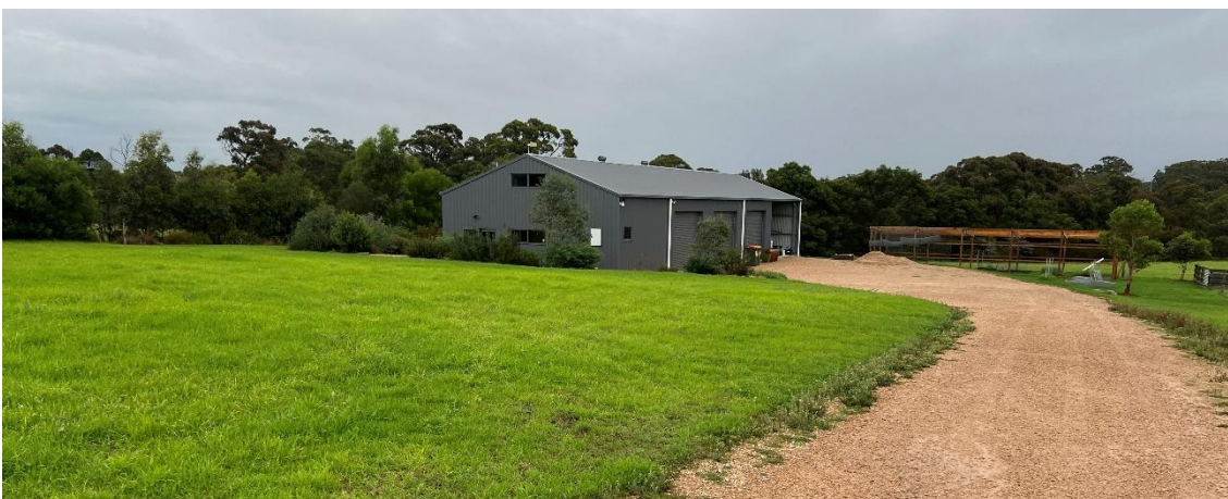
Image of the shed on the subject land partly used as a dwelling
