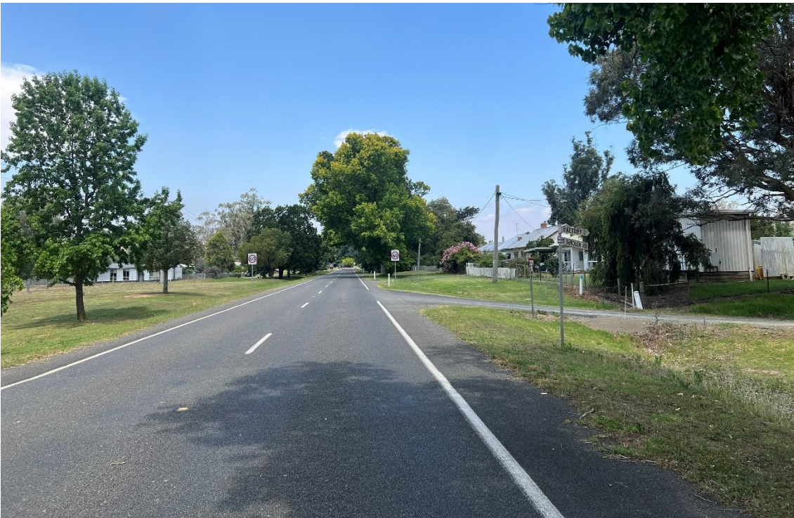
Looking north-west along Great Alpine Road from intersection with Factory Lane
