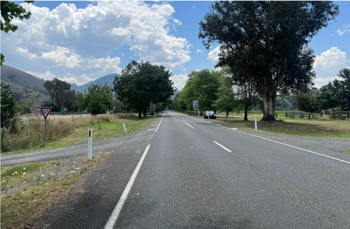
Looking north-west along Great Alpine Road from intersection with Factory Lane
