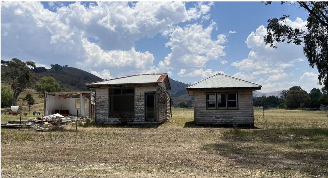
Aged structures on the subject land, viewed from south-eastern section of Factory Lane
