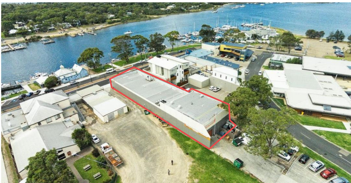
Figure 2 - Building Subject to Development (former 'Foodworks' Site)
