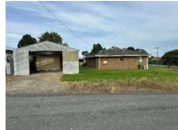
Photograph 7 – Existing carport on the northern boundary facing south.
