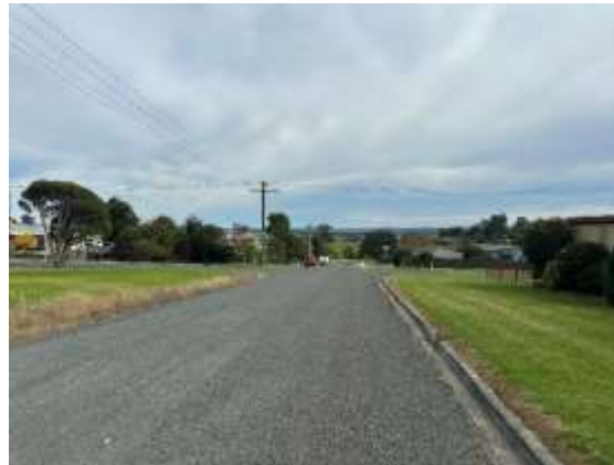
Photograph 17 – Stanley Street, facing west.
