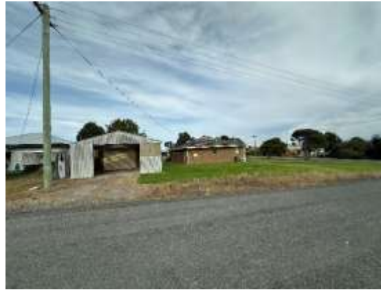
Photograph 10 – Location of proposed Unit 3 facing south.
