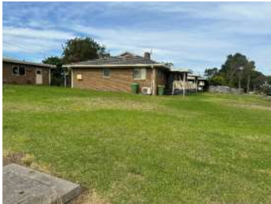
Photograph 9 – Location of proposed Unit 3 facing southeast.
