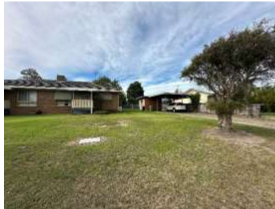
Photograph 11 – Location of proposed Unit 4 facing east.
