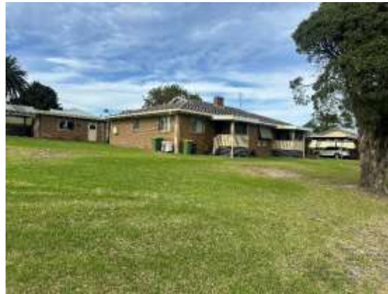
Photograph 5 – Location of proposed concrete access on the northern portion of the western boundary.
