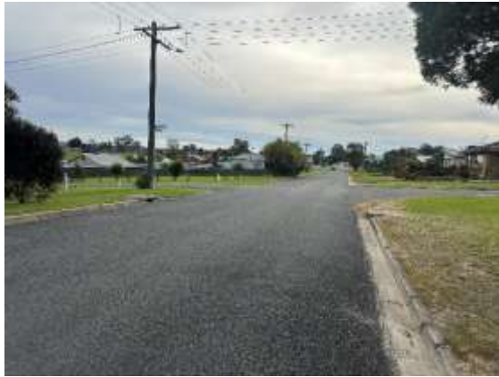
Photograph 14 – Gordon Street, facing north.
