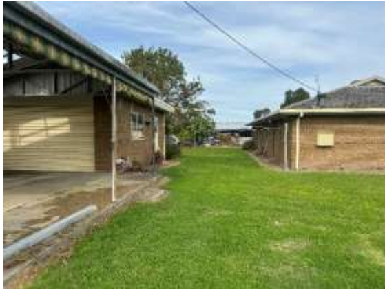
Photograph 8 – Existing outbuilding on the eastern portion subject site facing south.
