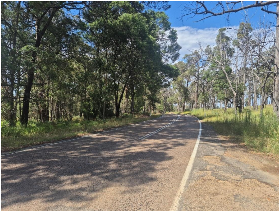
Looking south along Bullumwaal Road from existing access
