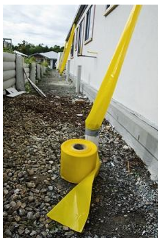
Figure 2 - Temporary Downpipes
