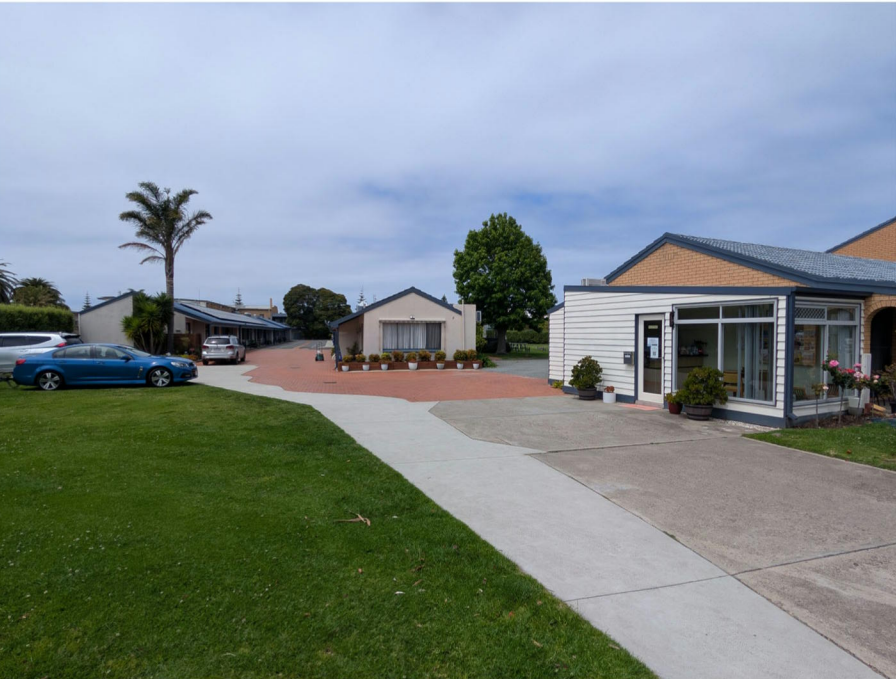
V4 ENTRY VIEW OF LAKESIDE MOTEL WATERFRONT BLOCK C, BLOCK D, OFFICE & BLOCK A (FROM LEFT TO RIGHT)
