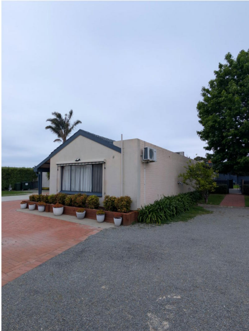
V7 NORTHERN VIEW OF BLOCK D
