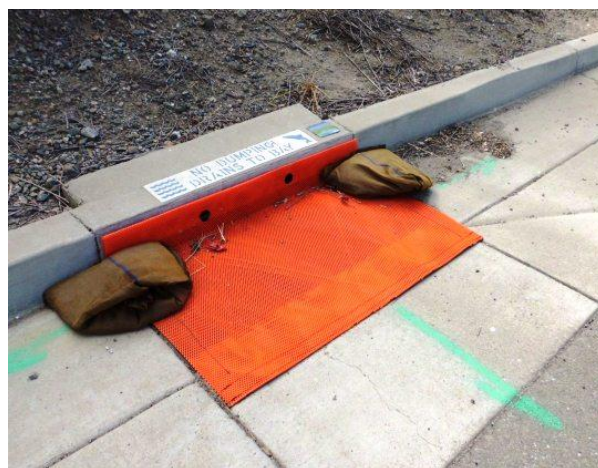
Figure 3 - Sediment Trap
