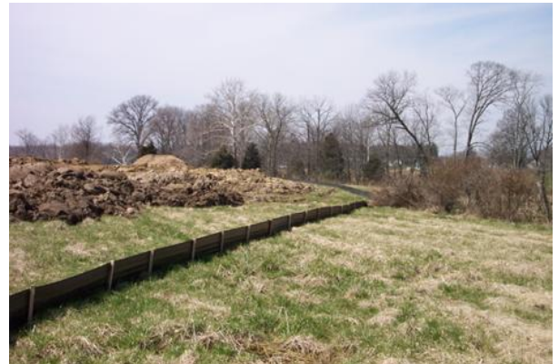
Figure 7 - Silt Fence (US EPA 2008)
