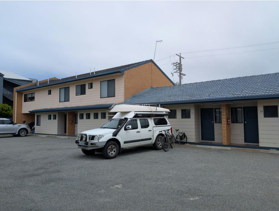
V9 SOUTHERN VIEW OF BLOCK A LEVEL 1 CARETAKERS RESIDENCE (TO BE DEMOLISHED)
