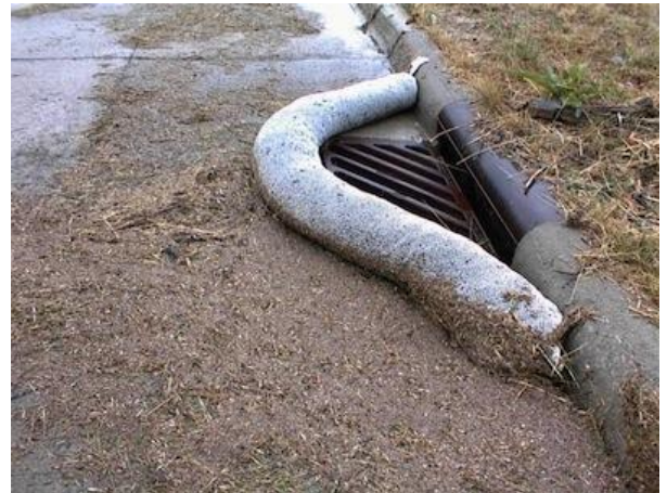
Figure 5 - Sediment Trap
