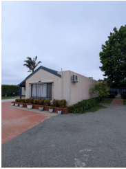
V7 NORTHERN VIEW OF BLOCK D
