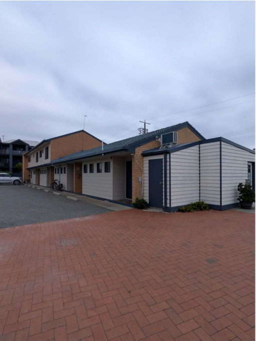
V8 EASTERN VIEW OF OFFICE & BLOCK A VIA DRIVEWAY
