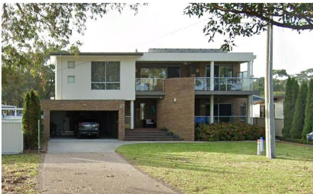
47 Jorgensen Street (Source: Google Earth)
