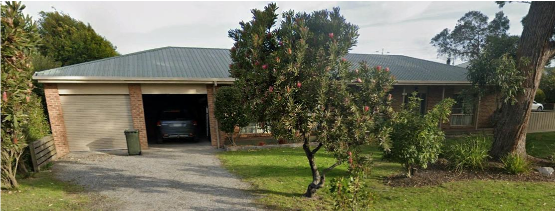
28 Rodwell Street from Jorgensen Street (Source: Google Earth)
