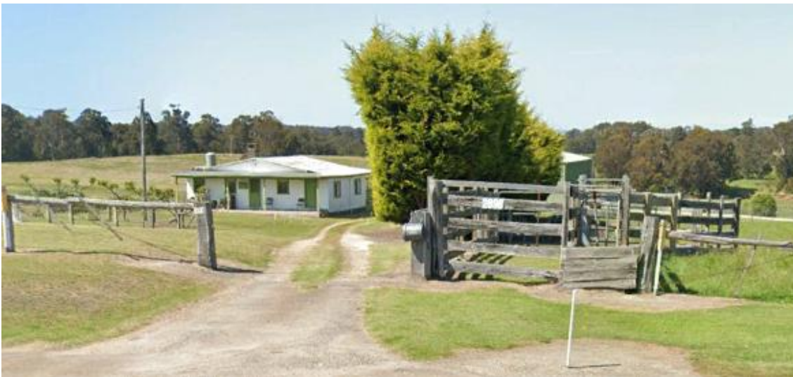
Existing dwelling and cattle yards in poor condition (Source: Google Earth)
