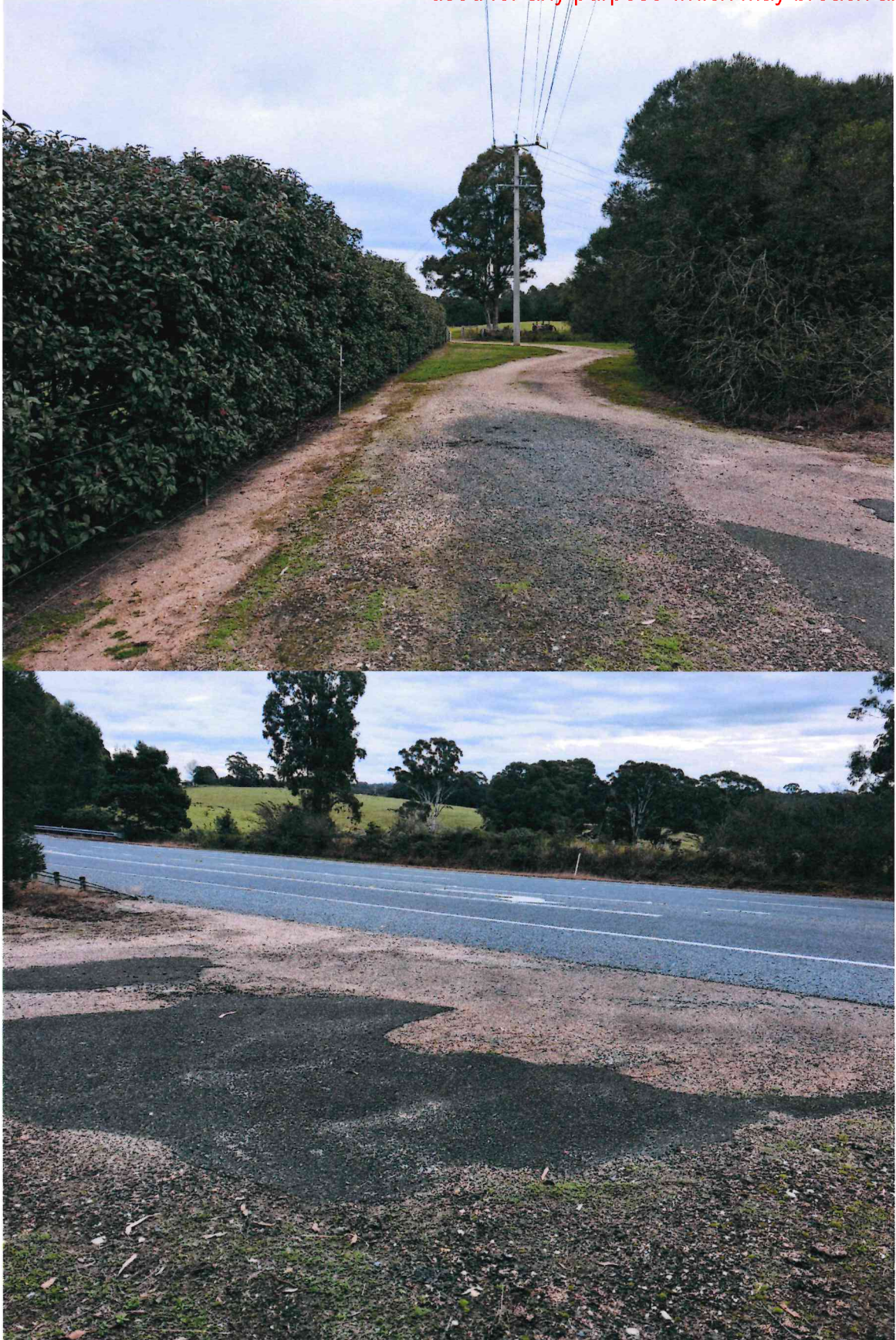
Photos of accesses to both properties.
