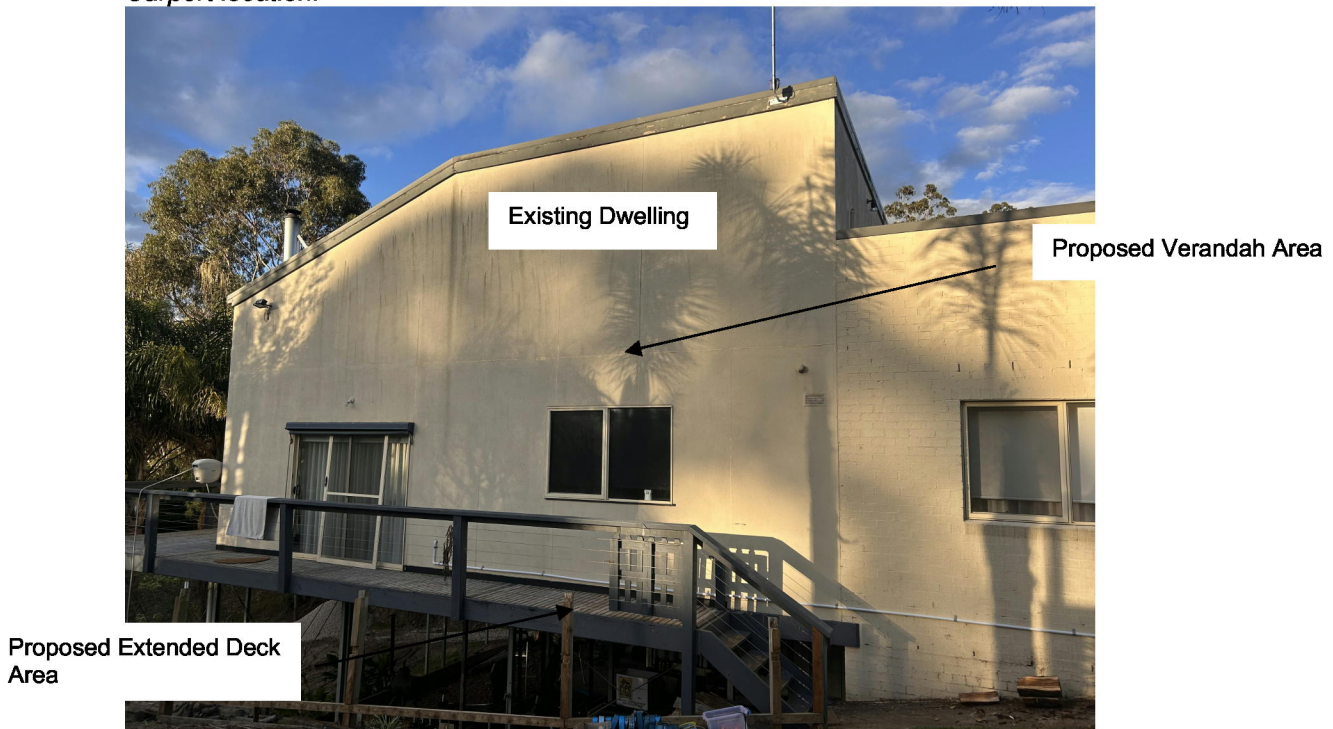
Photo Above - Photo from the West side boundary of the allotment looking East onto the Existing Dwelling and Proposed Verandah area.
