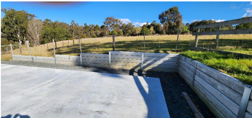
Figure 3 - Existing Concrete Retaining Wall
