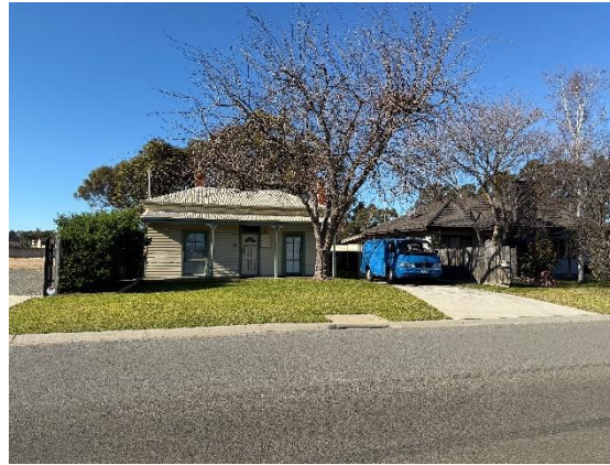
Photograph 10 – Property adjoining the southwest at 18 Hadfield Street, Lucknow.
