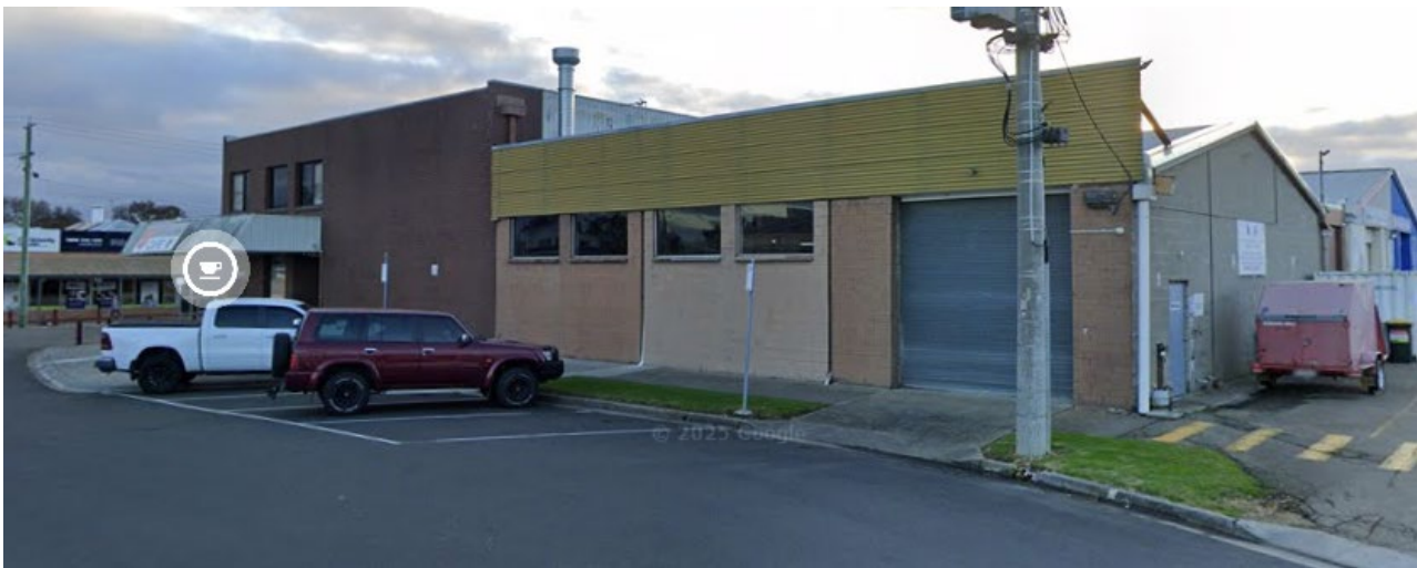
Figure 7 - Google Streetview image of site frontage to Bailey Street
