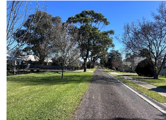
Photograph 12 – McKenzie Street facing west.
