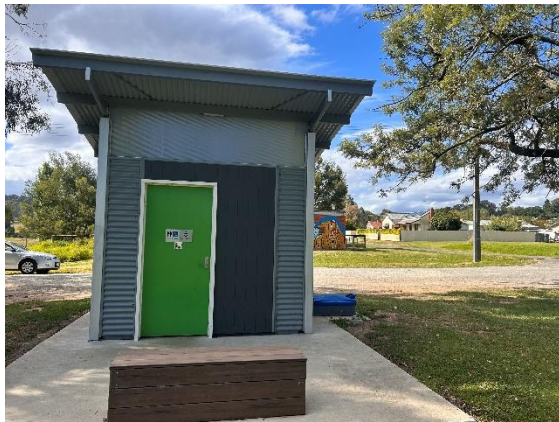
Photograph 15 – Bruthen Lions and Skate Park existing toilet amenities adjoining the southern boundary.
