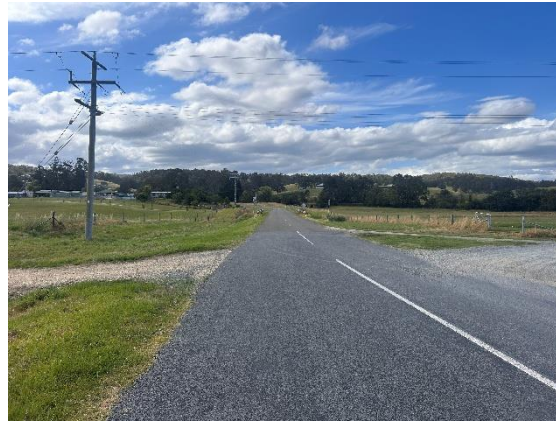
Photograph 16 – Station Road facing north.
