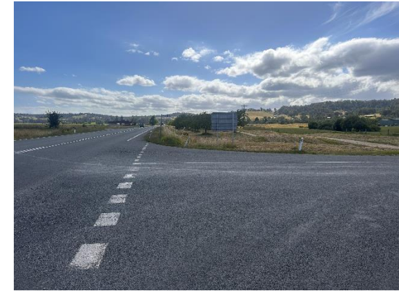
Photograph 18 – Intersection between Great Alpine Road and Station Road facing west.
