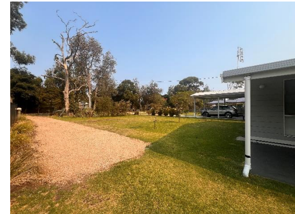
Photograph 7 – Location of proposed additions adjoining the eastern side of the existing dwelling facing southeast.
