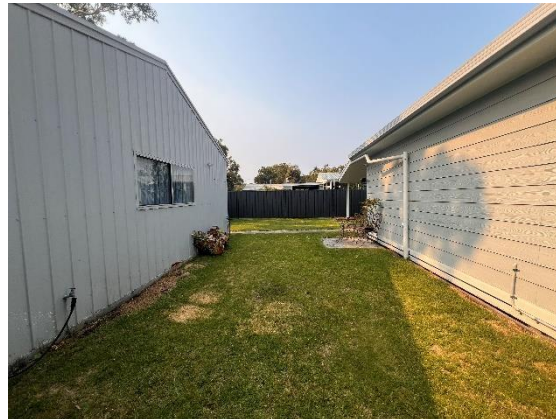
Photograph 5 – Location of proposed additions adjoining the western side of the existing dwelling facing north.
