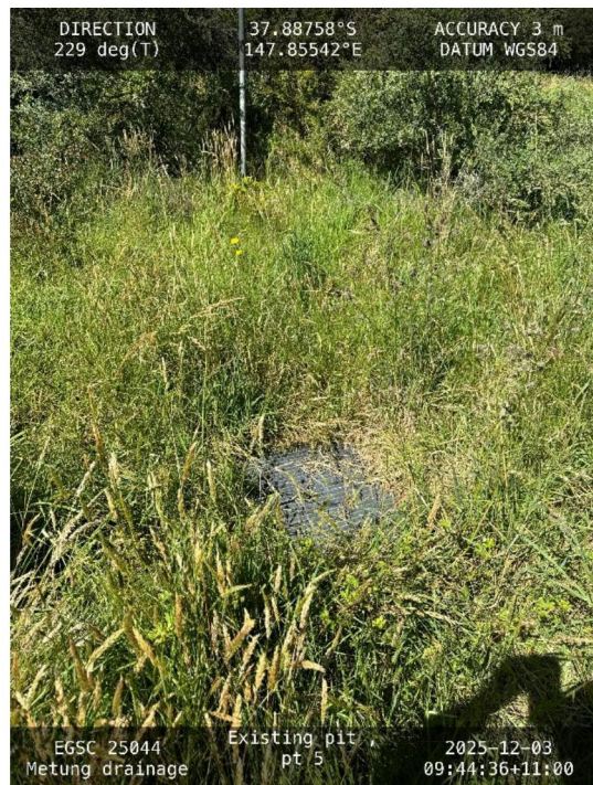
Plate 6. Weedy area around an existing stormwater pit.
