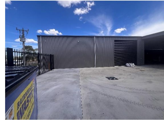
Photograph 6 – Subject site facing south.
