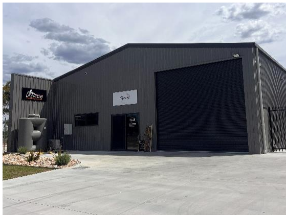
Photograph 3 – Existing industrial building and signage on subject site facing southwest.
