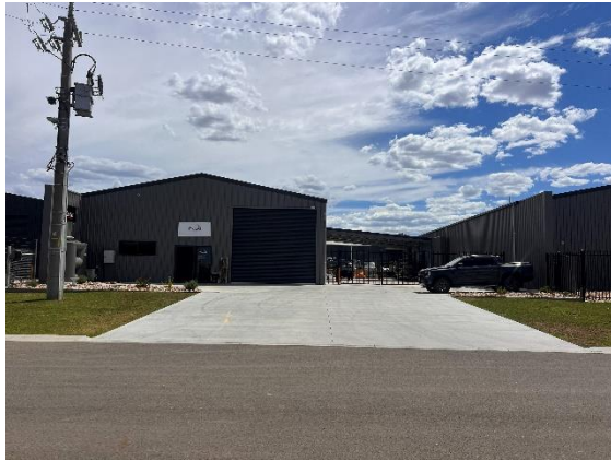
Photograph 2 – Subject site and existing crossover at 10 Grose Lane, Bairnsdale.
