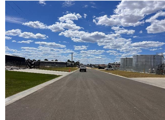
Photograph 12 – Grose Lane facing north.
