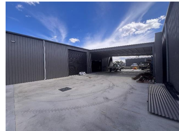
Photograph 7 – Subject site facing southwest
