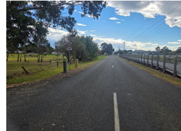
Photograph 12 – Lindenow-Glenaladale Road facing north.
