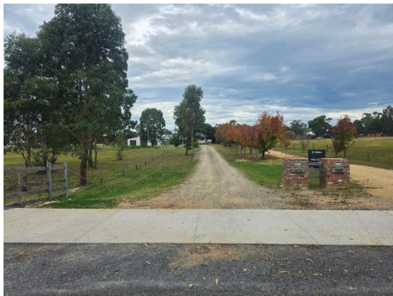
Photograph 3 – Existing crossover and driveway access to subject site.
