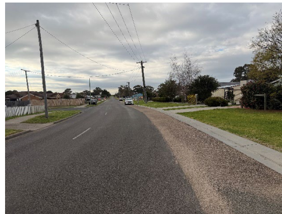
Photograph 17 – Crooke Street facing east at proposed Lot 2 location.
