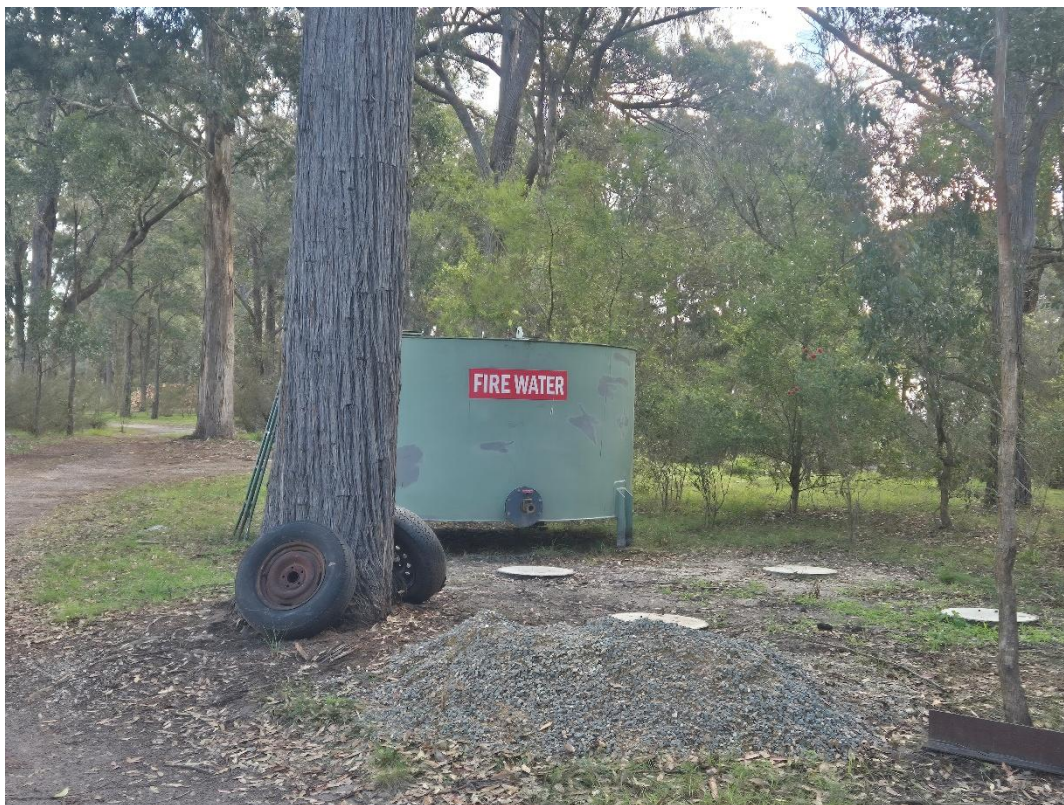
Existing water supply for fire fighting purposes
