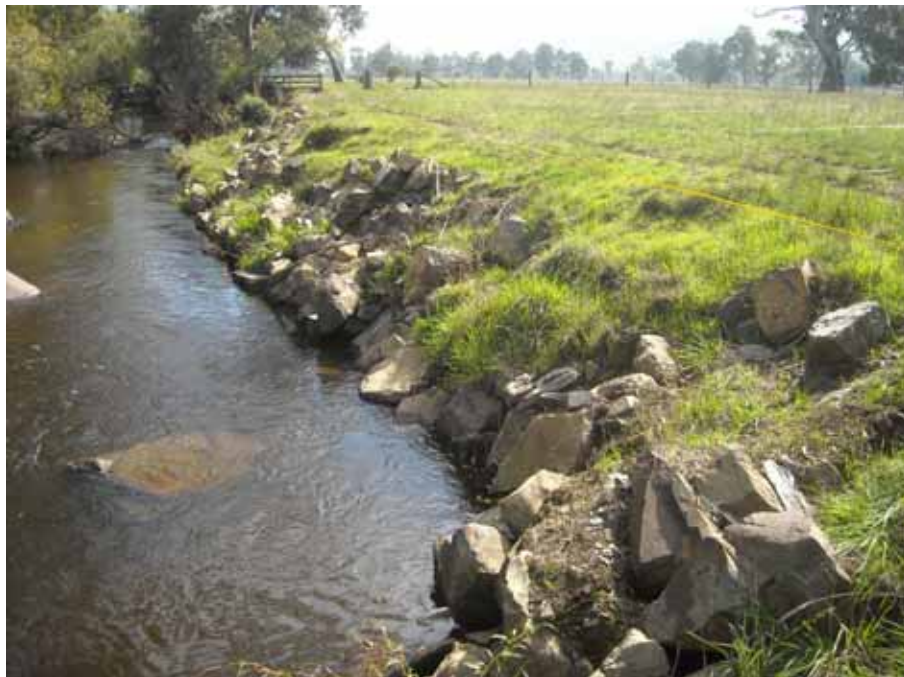
Figure 6-5 An example of rock beaching works
