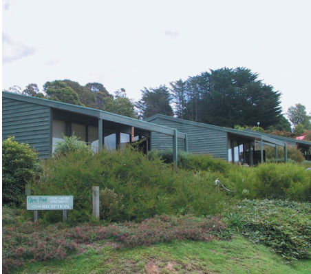
Gipsy Point accommodation overlooking the water
