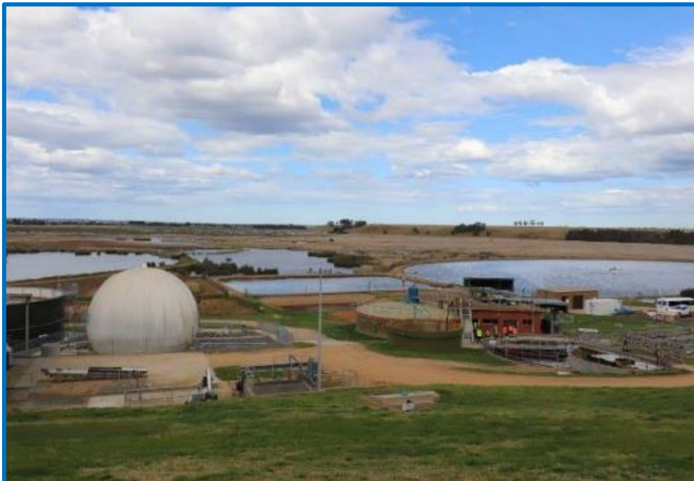
Bairnsdale Wastewater Treatment Plant
