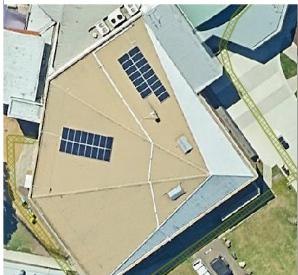
3. The Forge, 10kW solar
