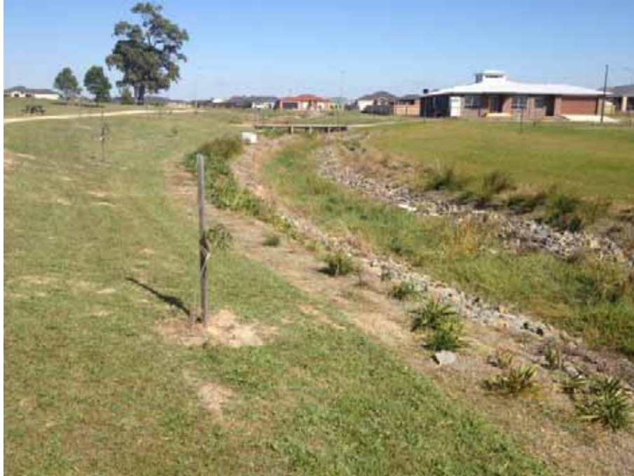
Figure 5-16 Stable formal drainage lines
