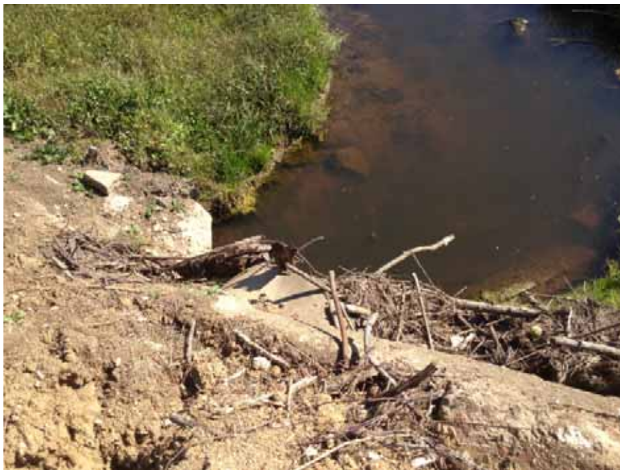
Figure 5-8 Temporary crossing barrier
