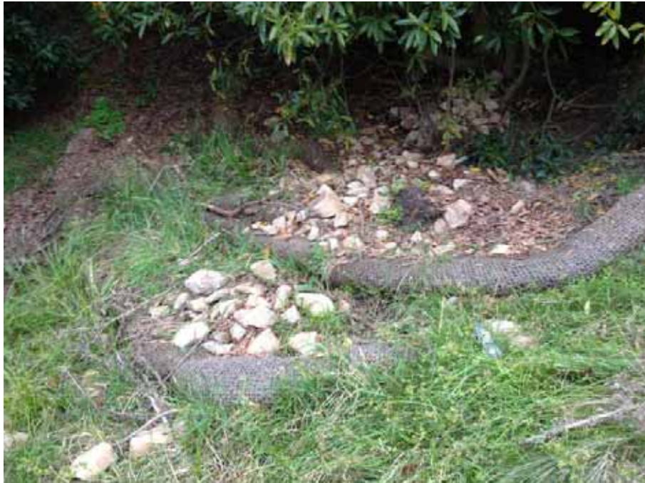
Figure 5-20 Stabilisation works with 'Eco-logs'
