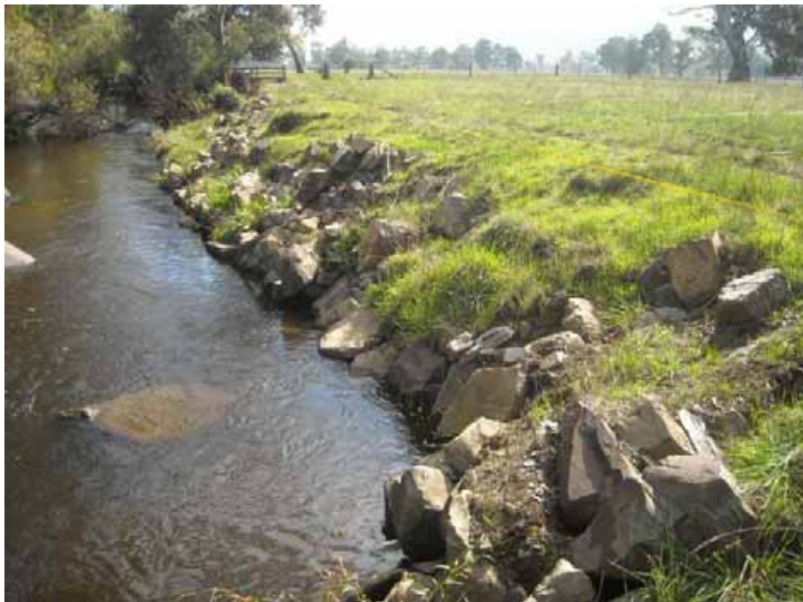
Figure 4-5 An example of rock beaching works
